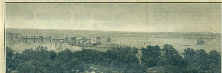
VIEW OF NATOMAS GREAT ROCK CRUSHING PLANT FROM FAIR OAKS.
